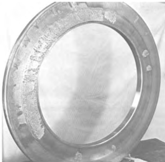
FIG. 4.1 (2342-28C) FAILURE INDUCED BY CORROSION
